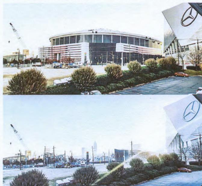
Nearly 5,000 pounds of explosives were used to bring down the Georgia Dome on Nov. 20 just after 7:30 a.m. The sound of the implosion could be heard all over Intown as the 25-year-old stadium collapsed.
